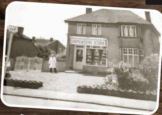
Carpenters Stores, Furnham Road.
