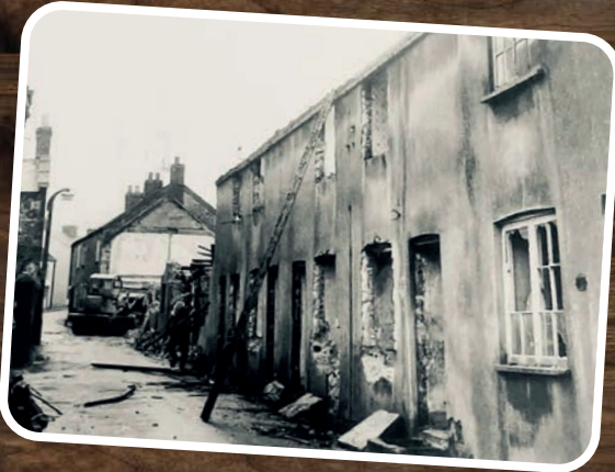
Demolition of Bath Street
